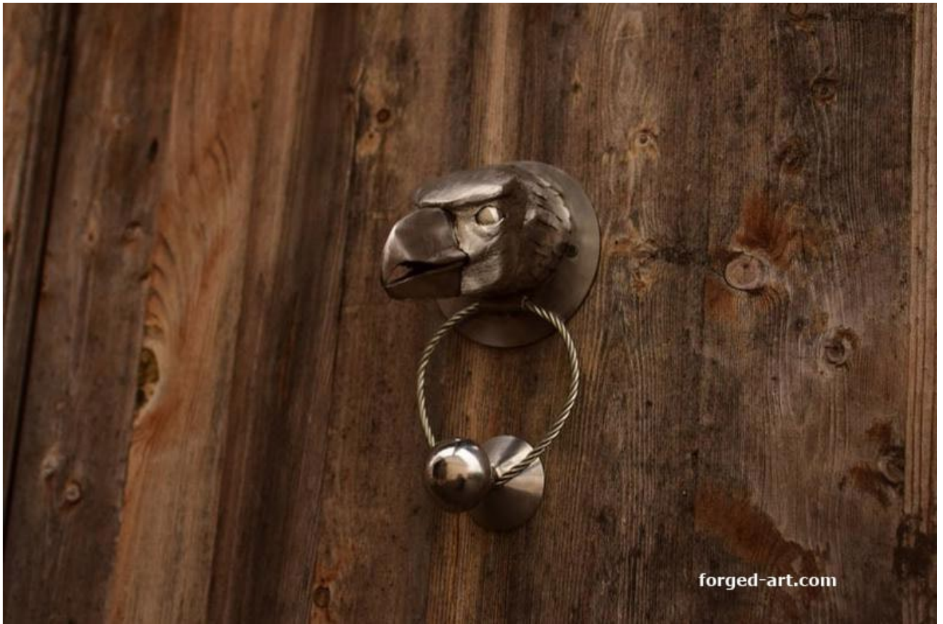
Hand knocker made of stainless steel
